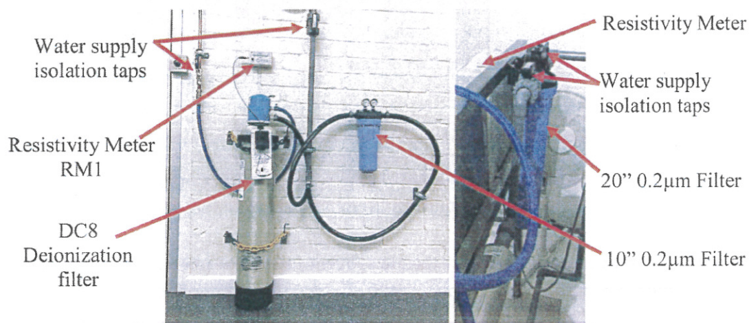
Figure 16: Location of the 0.2µm Filters and DC8 Filter.
