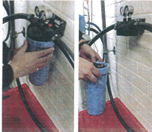
Figure 18: Removing the filter housing.
