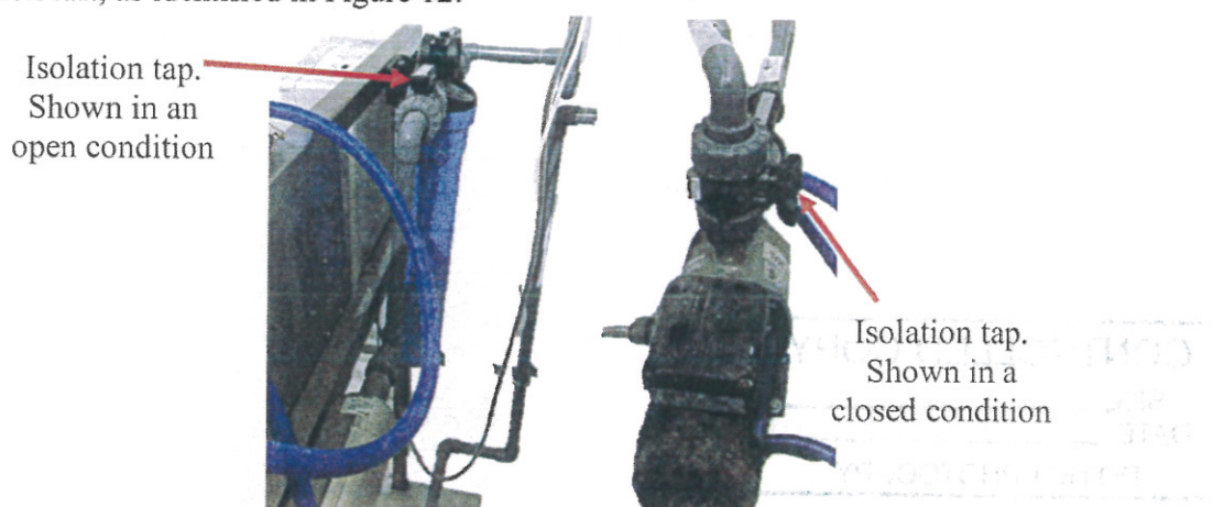
Figure 13: Location of the isolation taps.
