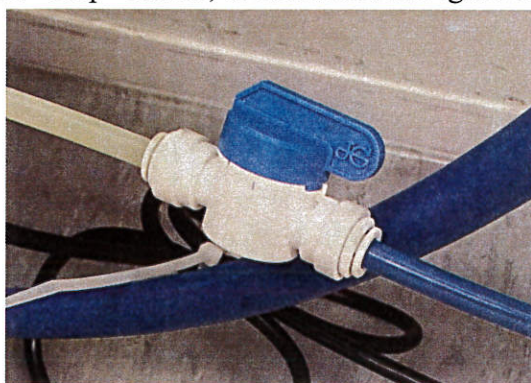
Figure 5: Top up adjuster shown a fully open condition, see Figure 1: For location.
